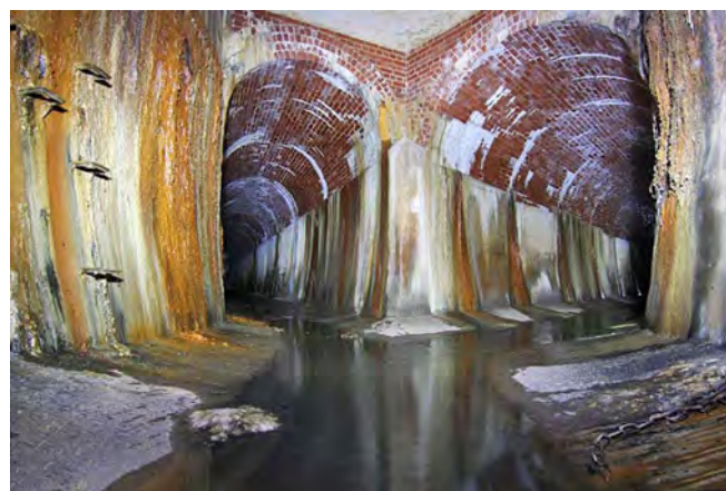
Sewer junction in the Markeaton Interceptor
